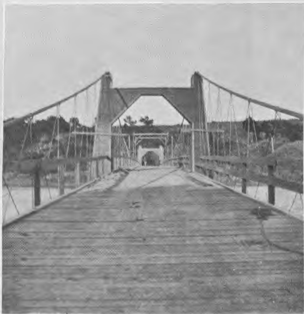
SUSPENSION BRIDGE 400 FEET LONG OVER SOUTH CANADIAN RIVER AT NOBLE.
