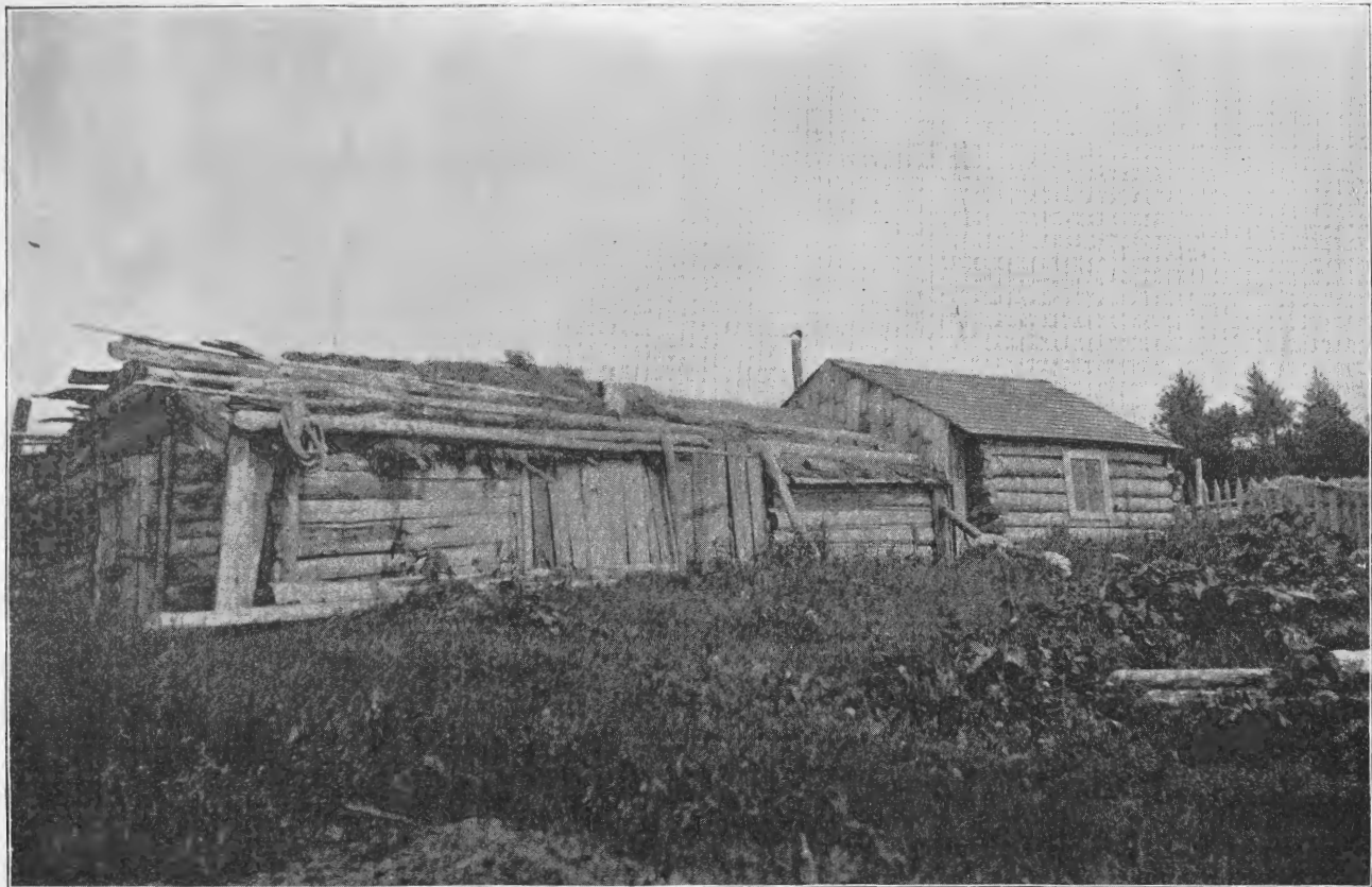
NATIVE BUILDINGS AT KADIAK.
